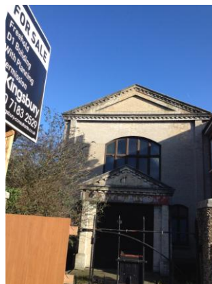
The former Christian Israelite church, Dames Road awaiting redevelopment
